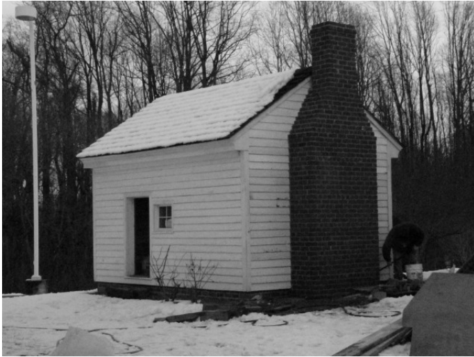
New chimney on slave quarters
