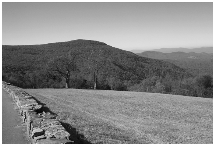
Walls constructed by CCC
