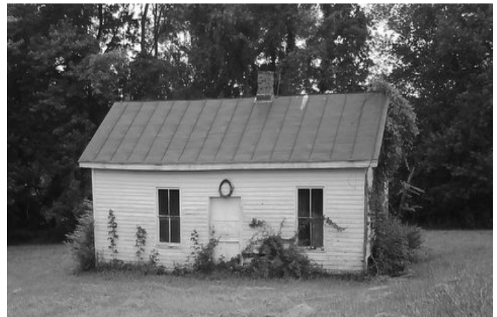
Newspaper building today
